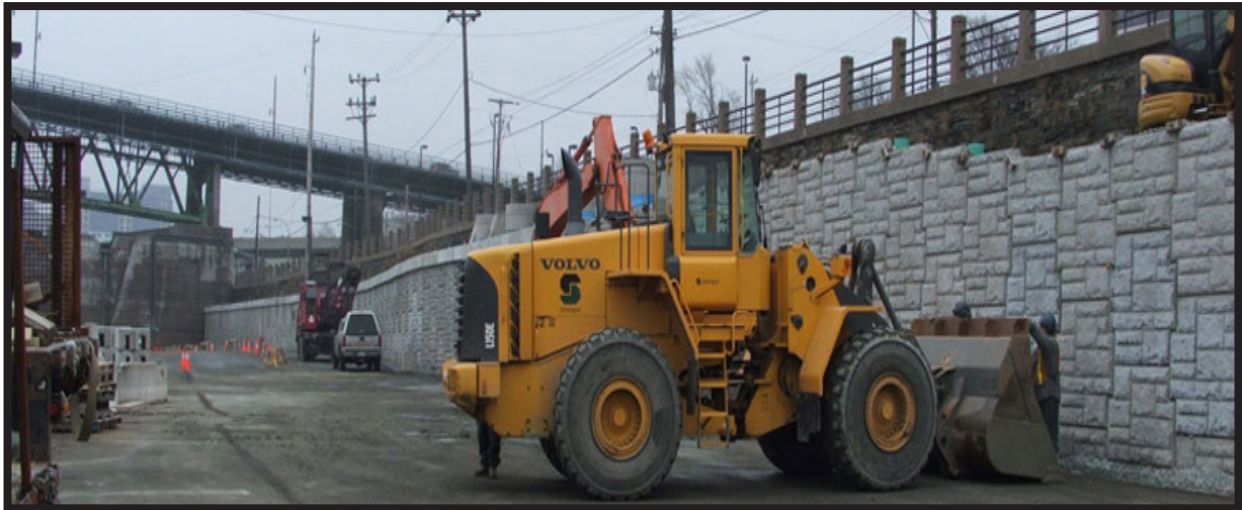
Figure 61: Photograph of the construction of the new retaining wall, 2016-2017. Construction of the new retaining wall in front of the old masonry wall from the 1870s. The rock bolts and pre-cut concrete blocks are visible. Where the current barrier lies, a concrete cap was fastened to the old masonry wall.
