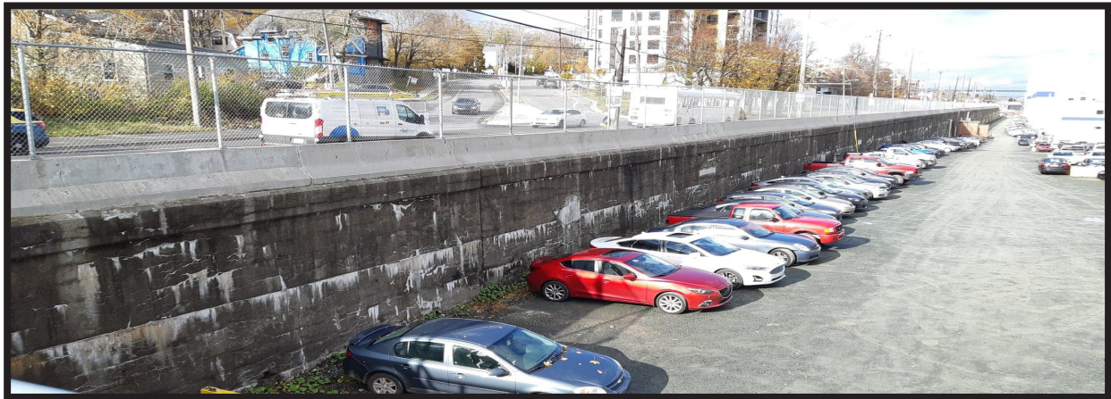
Figure : Photograph of the concrete retaining wall along the Irving Shipyards. (Source: Maenza, 2019)
